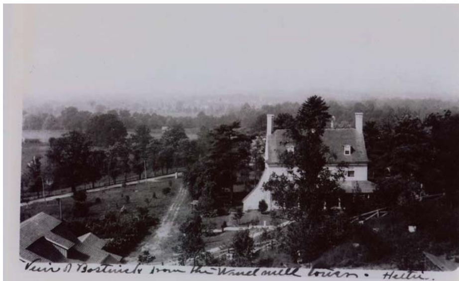
View of Bladensburg and Bostwick from a Watertower
