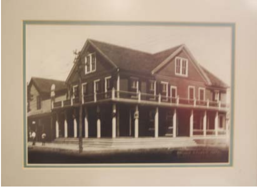
Josef Brown's Old House (Now Demolished) Alternate Rt. 1, Bladnesburg
