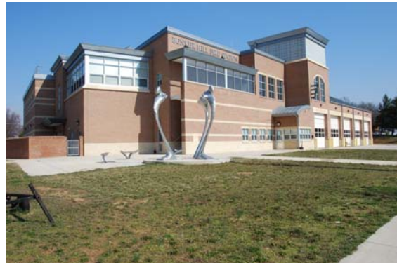
New Firehouse (Cottage City, Mt.Rainer, and Brentwood) Bunker Hill Fire Station
